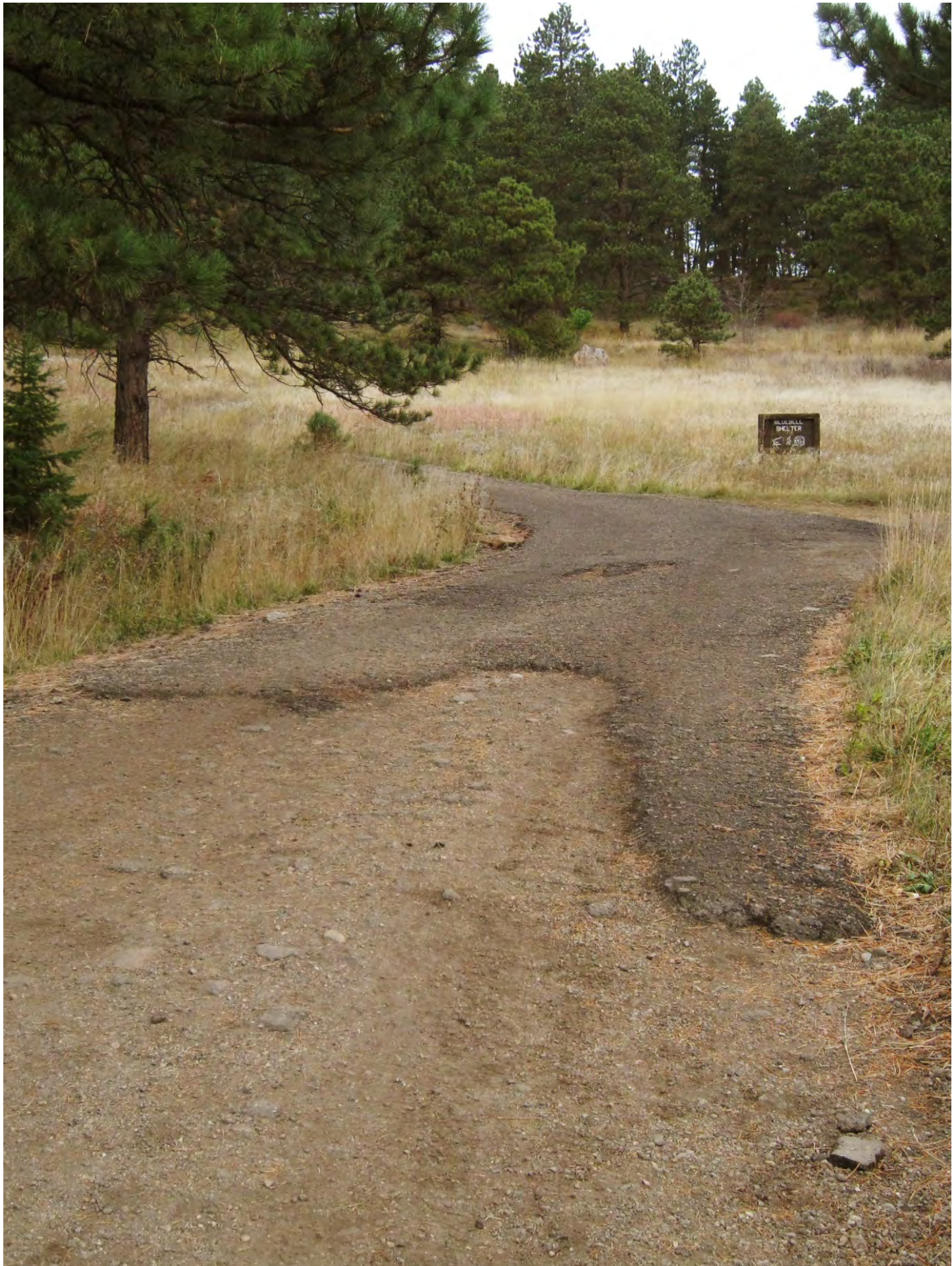
16 Deteriorating Asphalt on Bluebell Road
