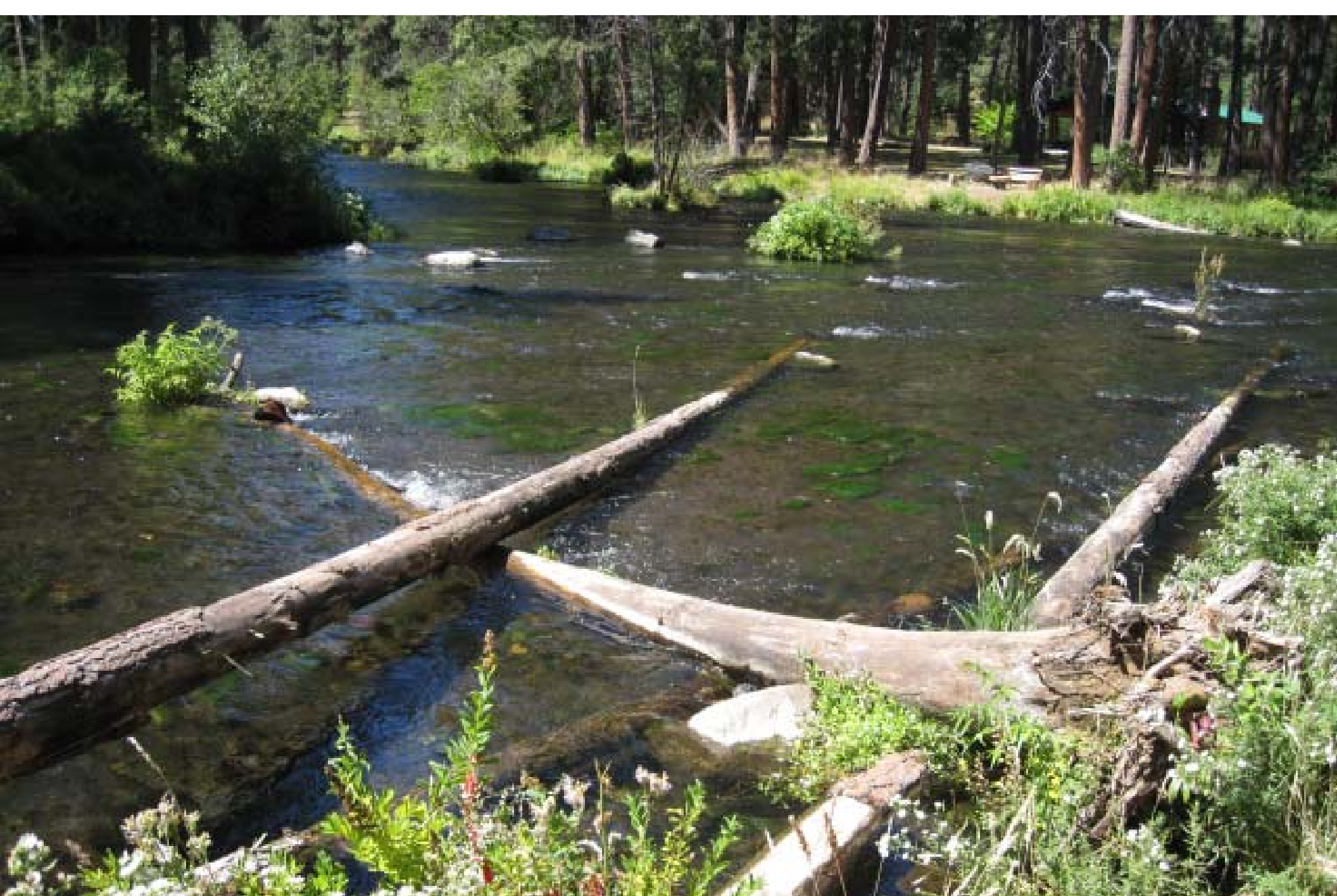
Metolius River Wood Restoration Project. A minimum of 4 pieces of wood per structure are recommended , as in this log jam across from the confluence with Spring Creek.
